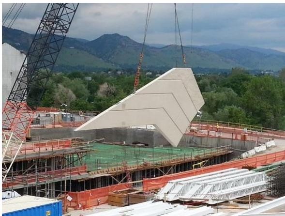
The majority of precast panels are 10" thick, with a composite design, and have 3" of Polyisocyanurate insulation at mid-depth of the wall panels.
